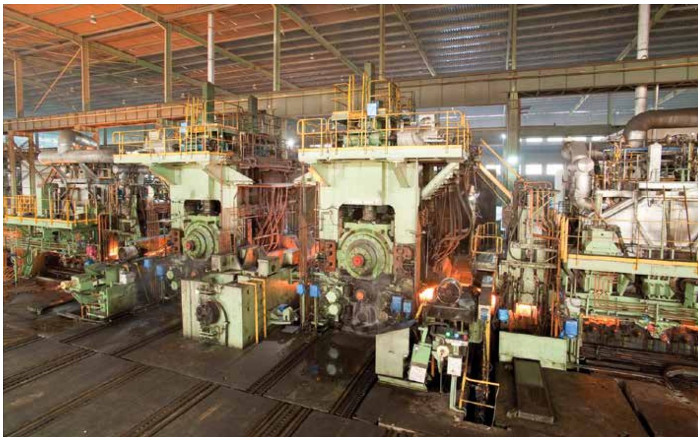
The centerpiece of a twin-stand Steckel mill is the millstands with the entry and exit-side Steckel furnaces in which the strip is heated between the reversing roll passes. The photo is the reference example of a comparable SMS plant
